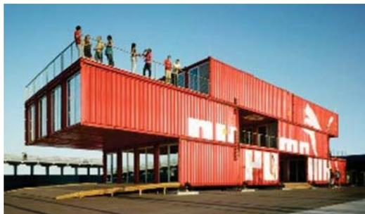
Shipping containers are used all over the world on trains, trucks, and especially on cargo ships. They come in two standard sizes: 8x8x20, or 8x8x40, making 160 or 320 square feet of space, which cost around \$1500 or \$2500 respectively. They have double doors on each end, and are constructed out of a steel frame with corrugated steel making the walls, floor, and ceiling.
